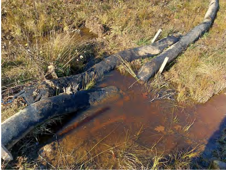
Silt sock floating with poor ground contact causing discharge to wetland
